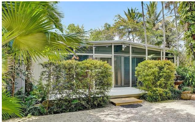
Existing Single-Family Residential Structure
