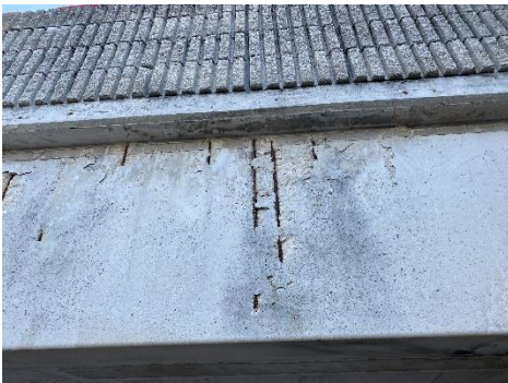
Exposed Rebar
