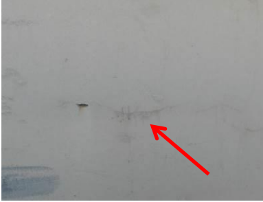
Figure 4: Fine Crack
