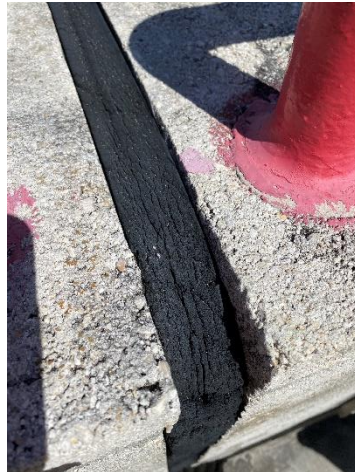
Vertical Expansion Joint
