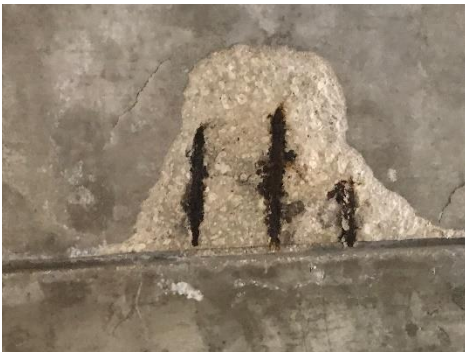
Exposed Rebar
