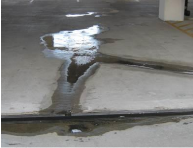
Figure 8: Ponding Water
