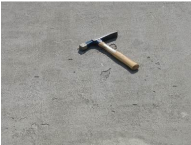
Figure 2: Concrete Delamination
