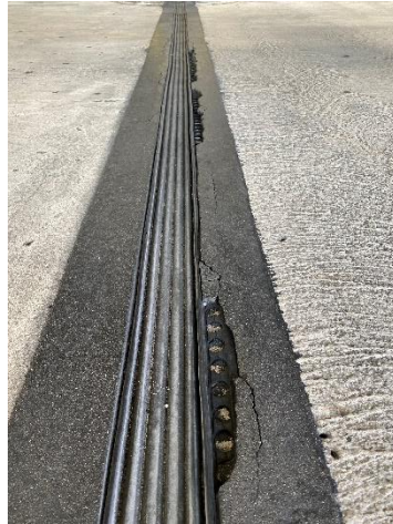
Horizontal Expansion Joint
