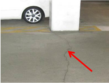
Figure 5: Medium Crack
