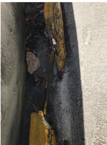
Damaged Curb
