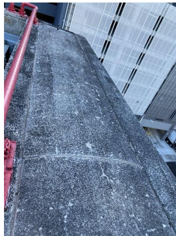
Horizontal Sealant at Planter
