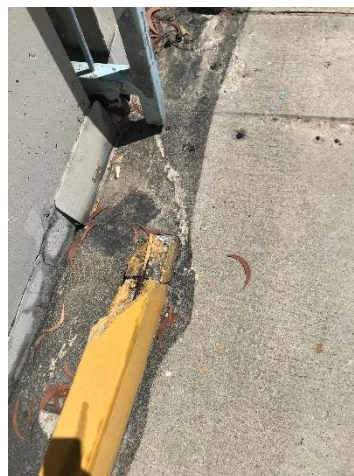
Damaged Curb
