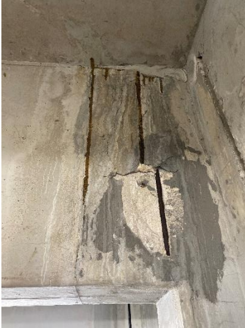
Exposed Rebar
