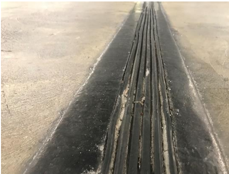
Horizontal Expansion Joint
