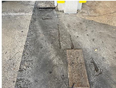
Exposed Rebar
