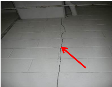
Figure 6: Wide Crack
