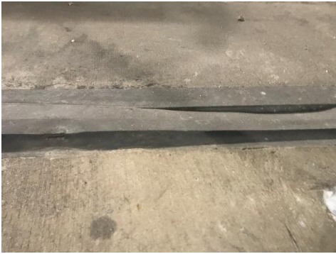
Horizontal Expansion Joint – Cover Plate
