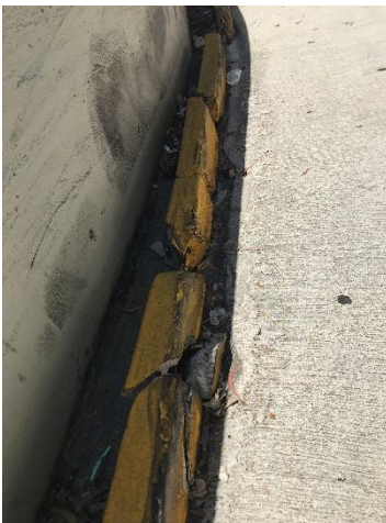
Damaged Curb
