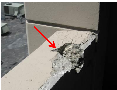
Figure 3: Concrete Spall
