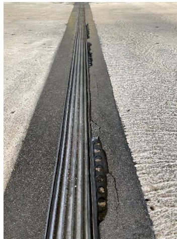
Horizontal Expansion Joint
