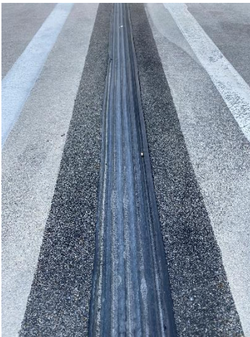
Horizontal Expansion Joint
