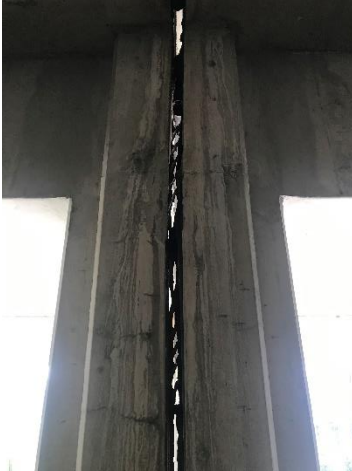
Vertical Expansion Joint
