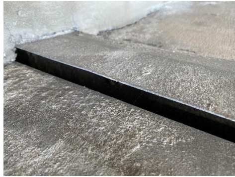
Horizontal Expansion Joint – Cover Plate
