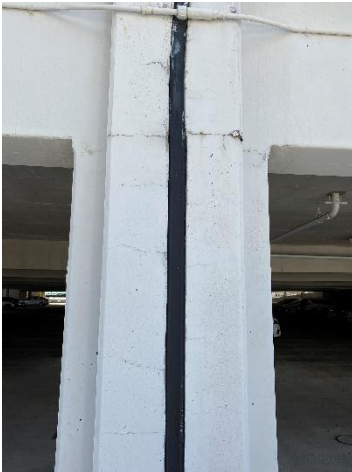
Vertical Expansion Joint
