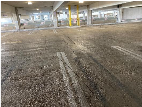
Floor Cracks
