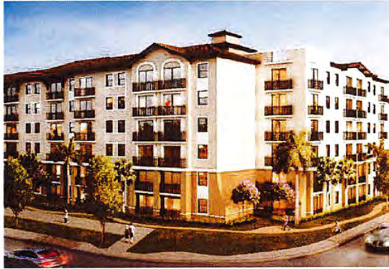
1 Arbor View (Margate/Affordable) 100 units completed in June 2018
