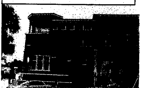
3031 Riomar Street 3-story townhouses
