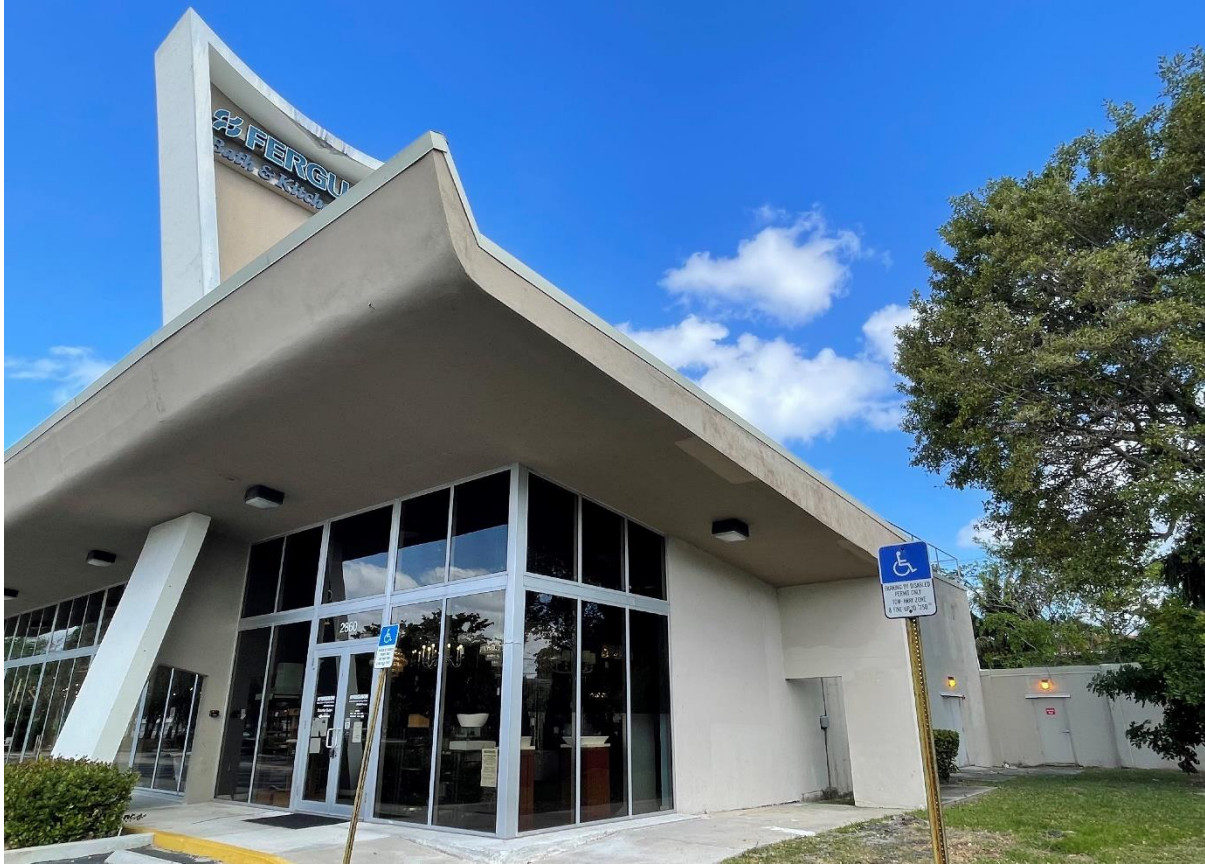
Front/South Elevation Looking Northeast
