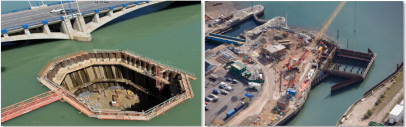
Exhibit 10 – Construction with Use of Cofferd Dam
