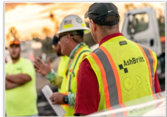
Safety management meeting prior to beginning work.
