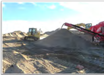
Sand Screening for Renourishment
