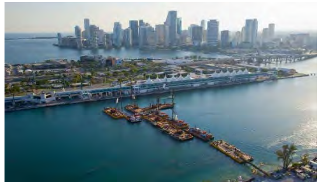
Channel ground improvement works on marine mode
