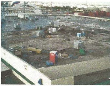
WIND MITIGATION & RE-ROOFING
