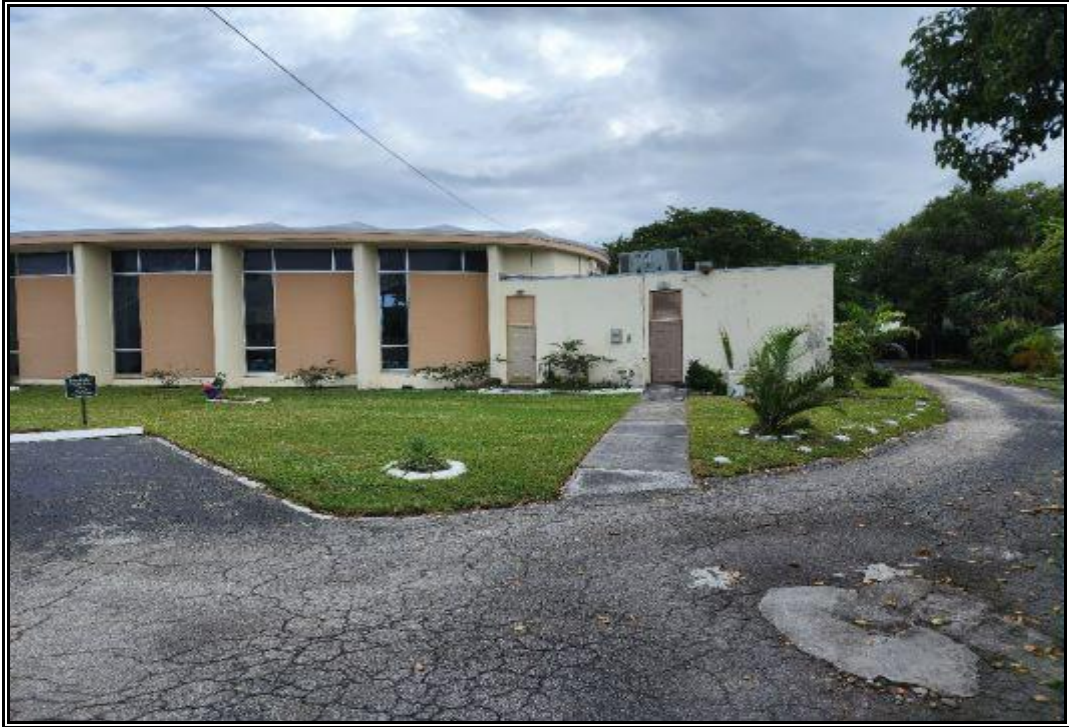
View of Subject property facing south
