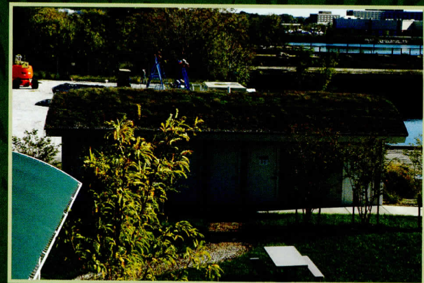
Port Covington. Green belts, right down to living roofs on some of the buildings, absorb rainwater before it gets to the bay, further preventing pollution.
