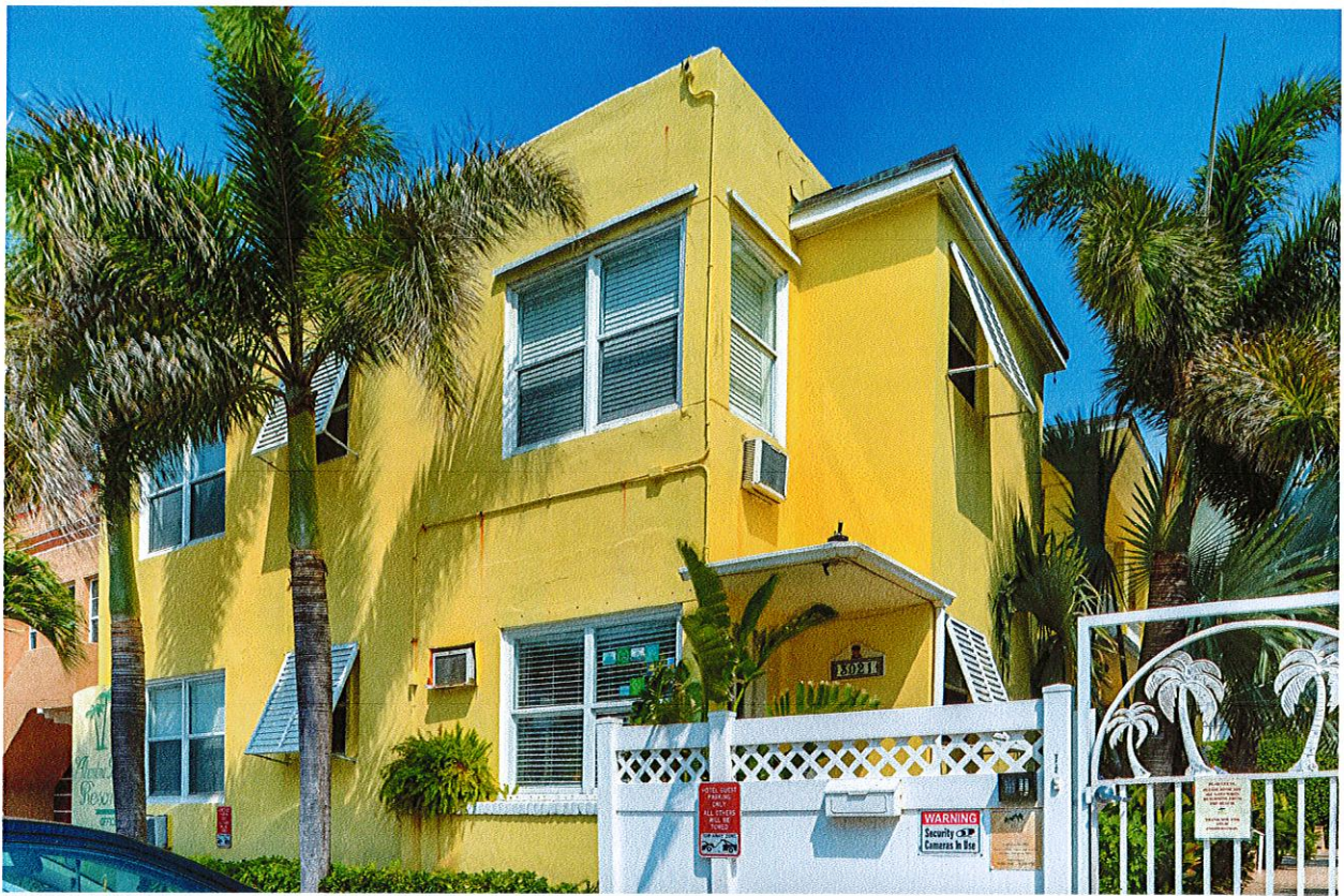
Southeast Corner showing projecting bathroom wing
