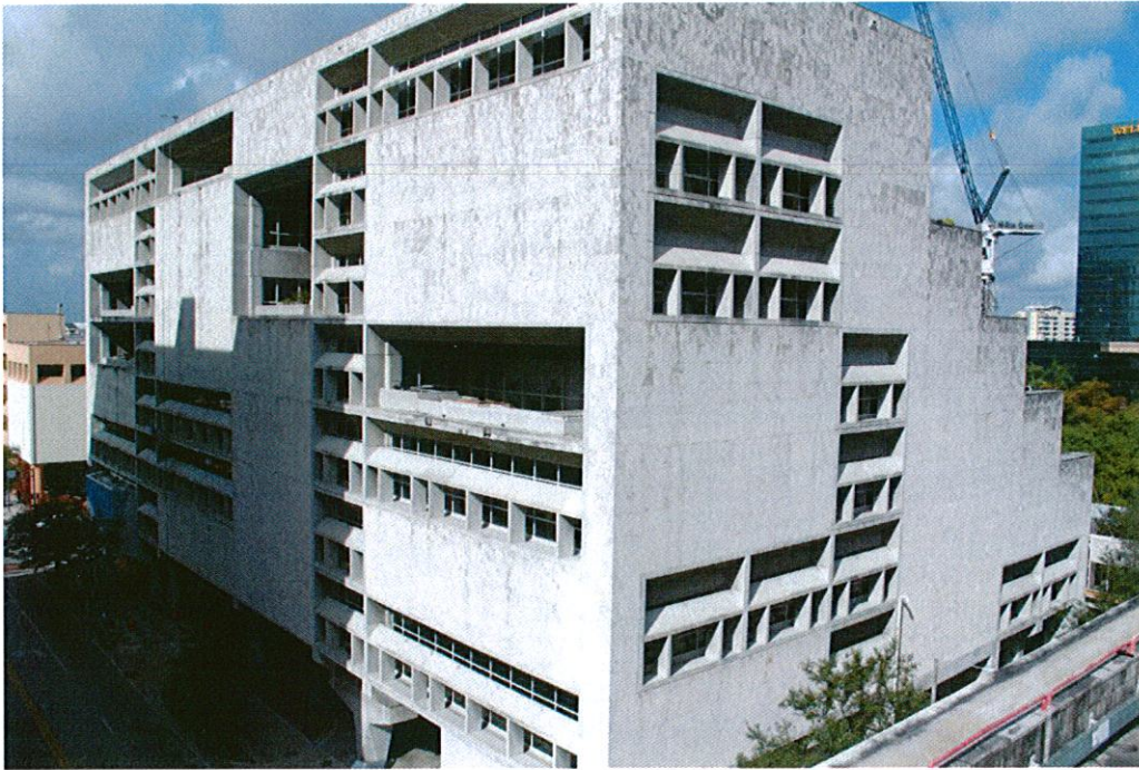
ABOVE: View of the east and south elevations. Note the integrated sun shades and the recessed terraces. RIGHT: View of the west elevation
