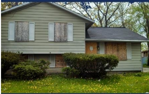
Current Plywood Board Up
