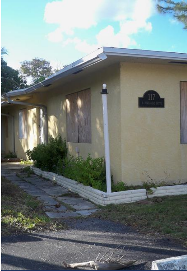
Current Plywood Board Up
