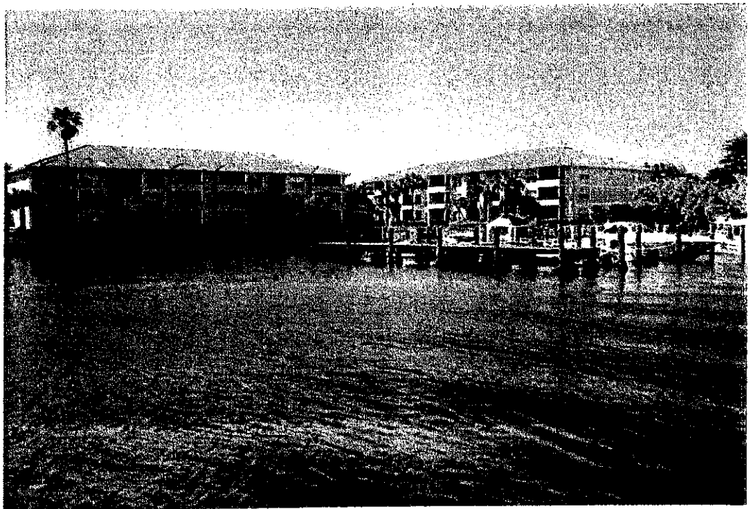
4. Northeastern portion of the basin, facing southwest.
