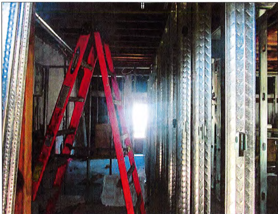
TENANT SPACE CURRENTLY UNDER CONSTRUCTION
