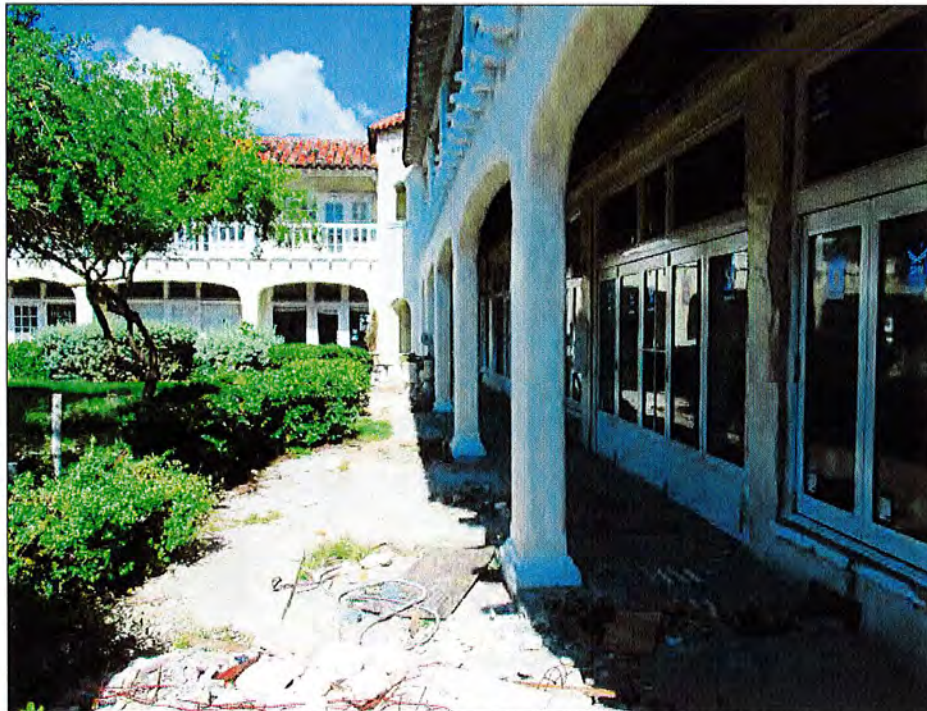
EXTERIOR VIEW OF TENANT SPACE CURRENTLY UNDER RENOVATION
