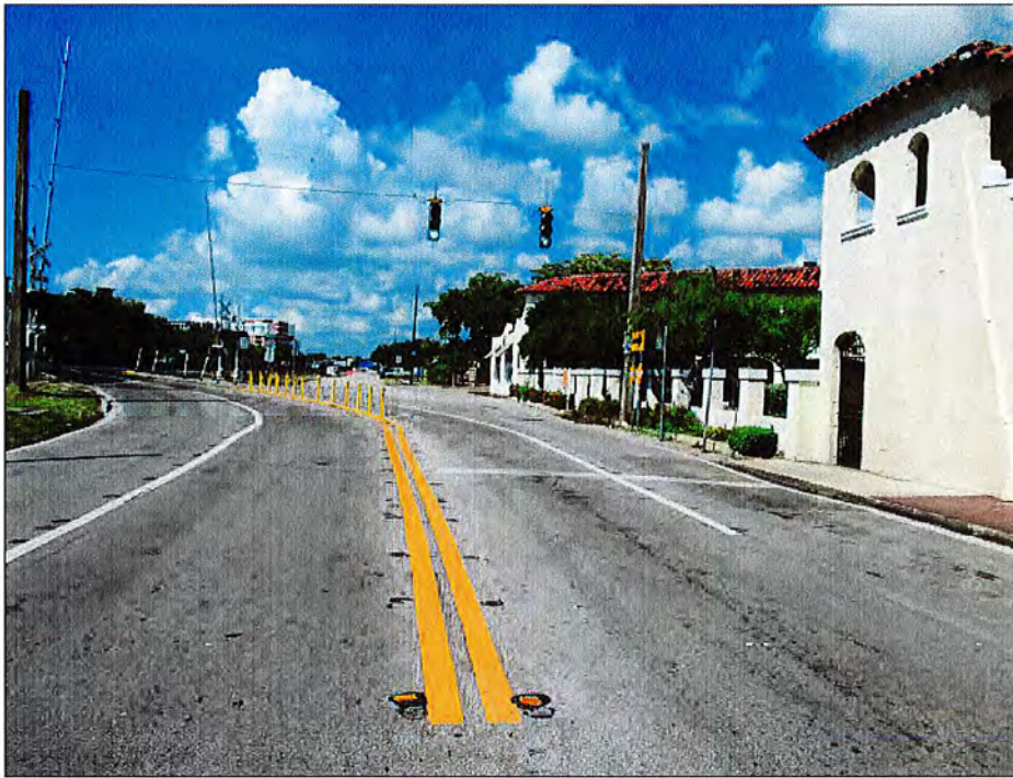
LOOKING SOUTH ALONG PROGRESSO DRIVE
