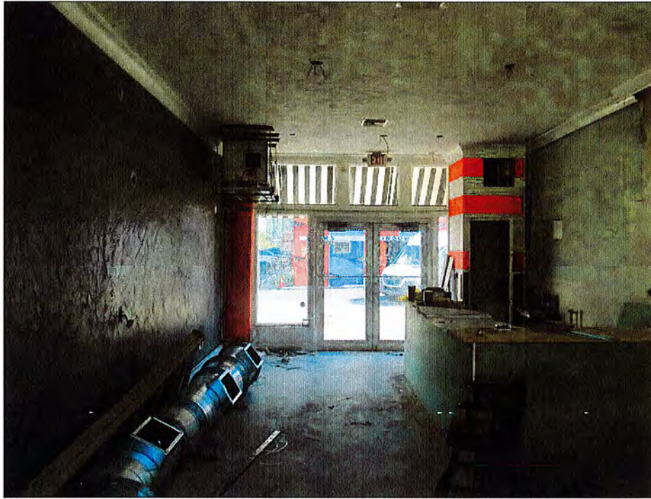
TENANT SPACE CURRENTLY UNDER CONSTRUCTION
