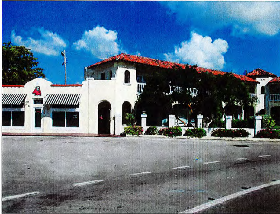
VIEW OF THE SUBJECT PROPERTY FROM PROGRESSO DRIVE
