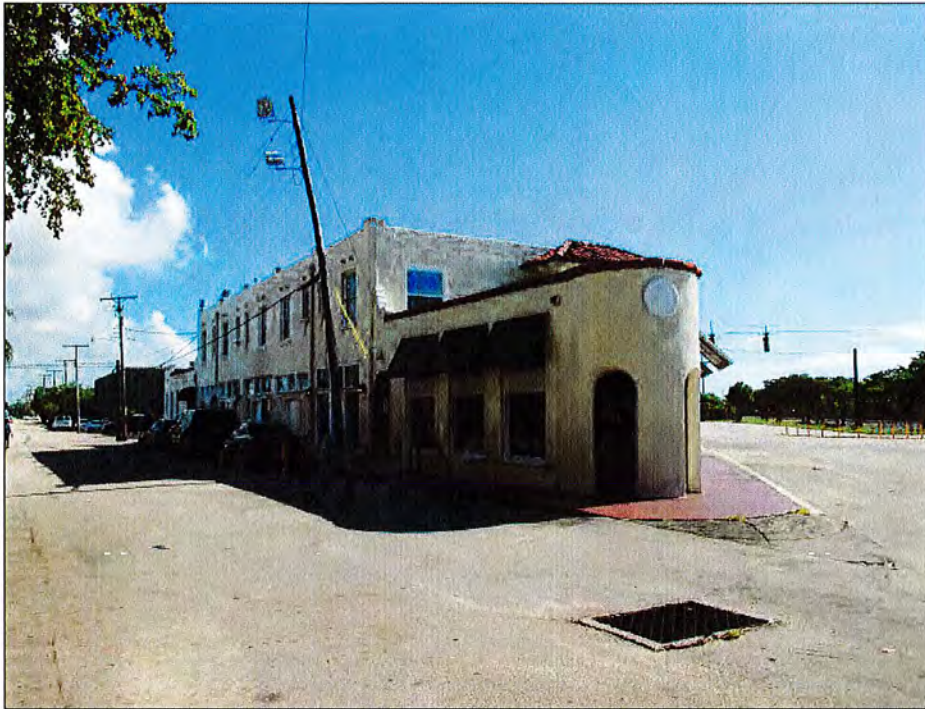
REAR VIEW OF THE SUBJECT PROPERTY FROM NE 3 RD AVENUE
