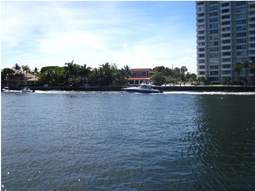
5. Northern Finger pier #3, facing southwest.
