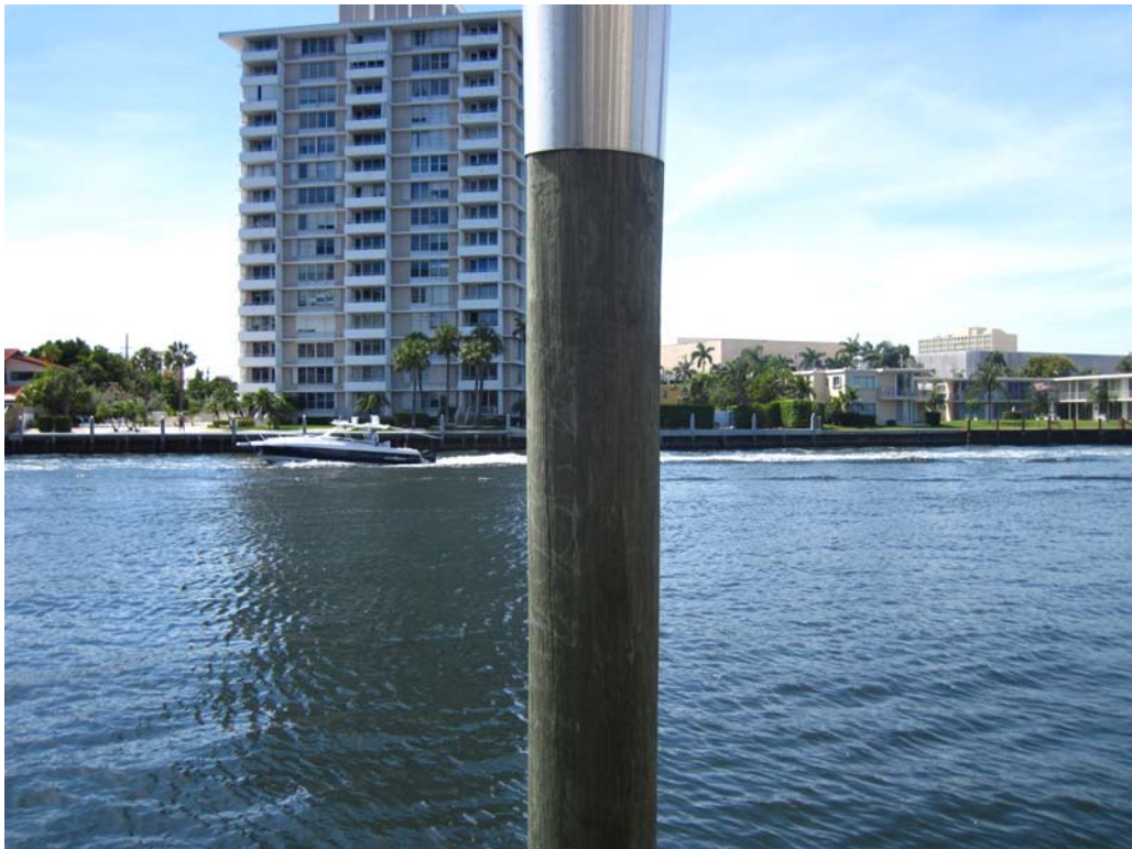
4. Northern Finger pier #3, facing west.
