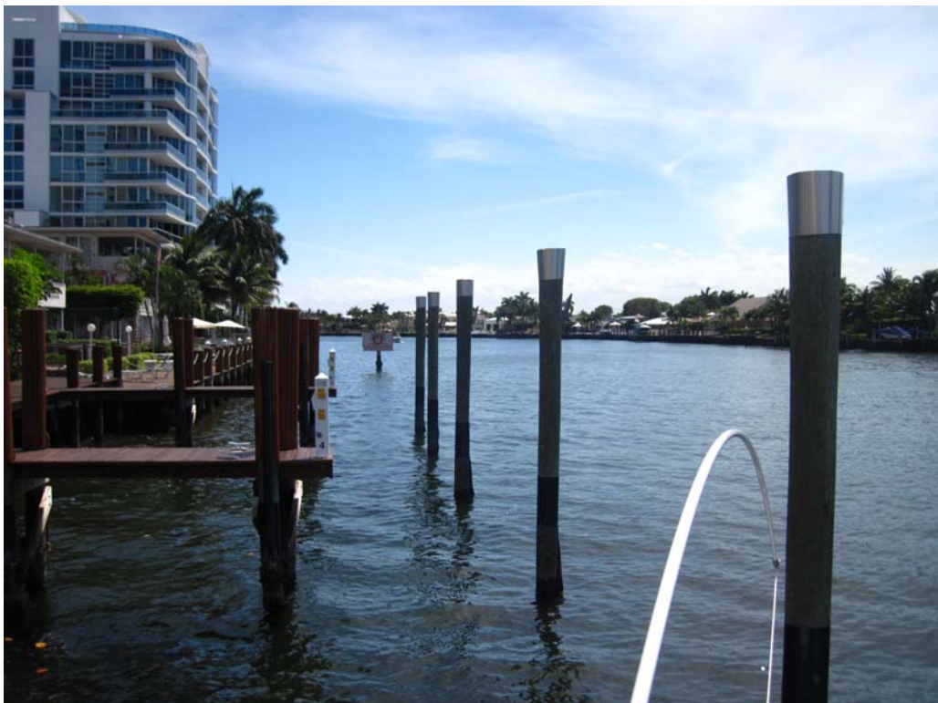
6. Northern Finger pier #3, facing south.
