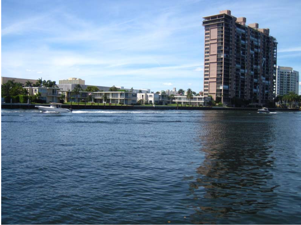
3. Northern Finger pier #3, facing northwest.
