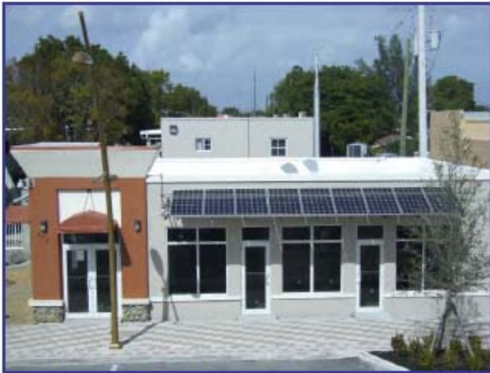
915 Sistrunk Boulevard, After
