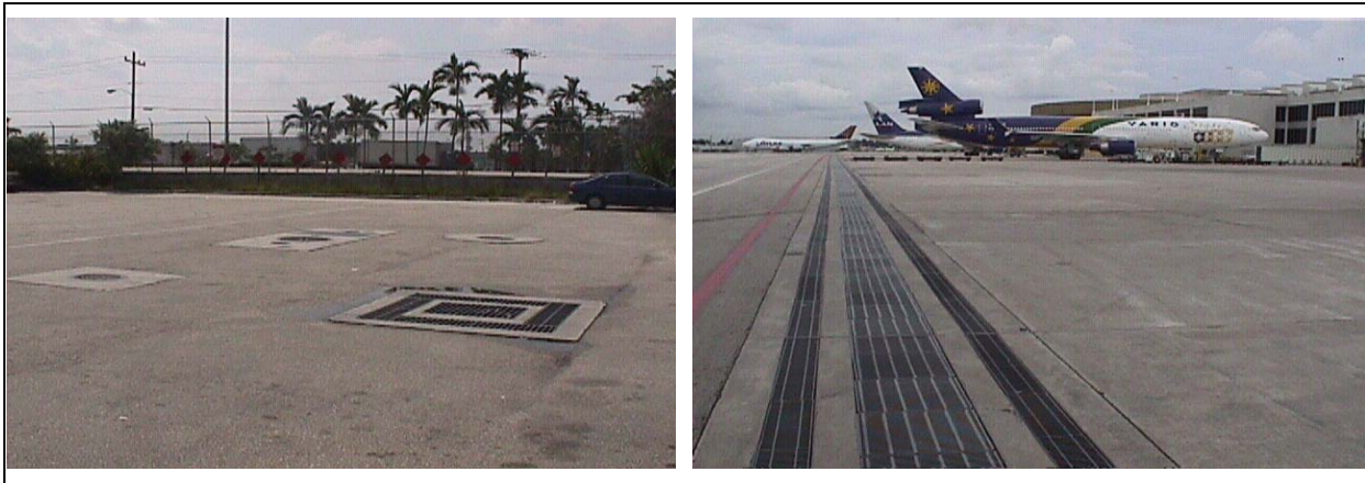
Figure 3-9: Photographs of First Flush Inlet Systems. (Source: Miami International Airport, MIA)
