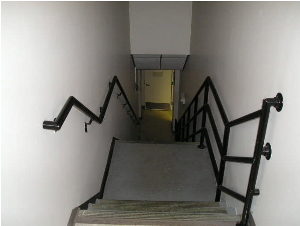
STAIRWAY TO 2ND FLOOR FROM NORTH SIDE ENTRANCE
