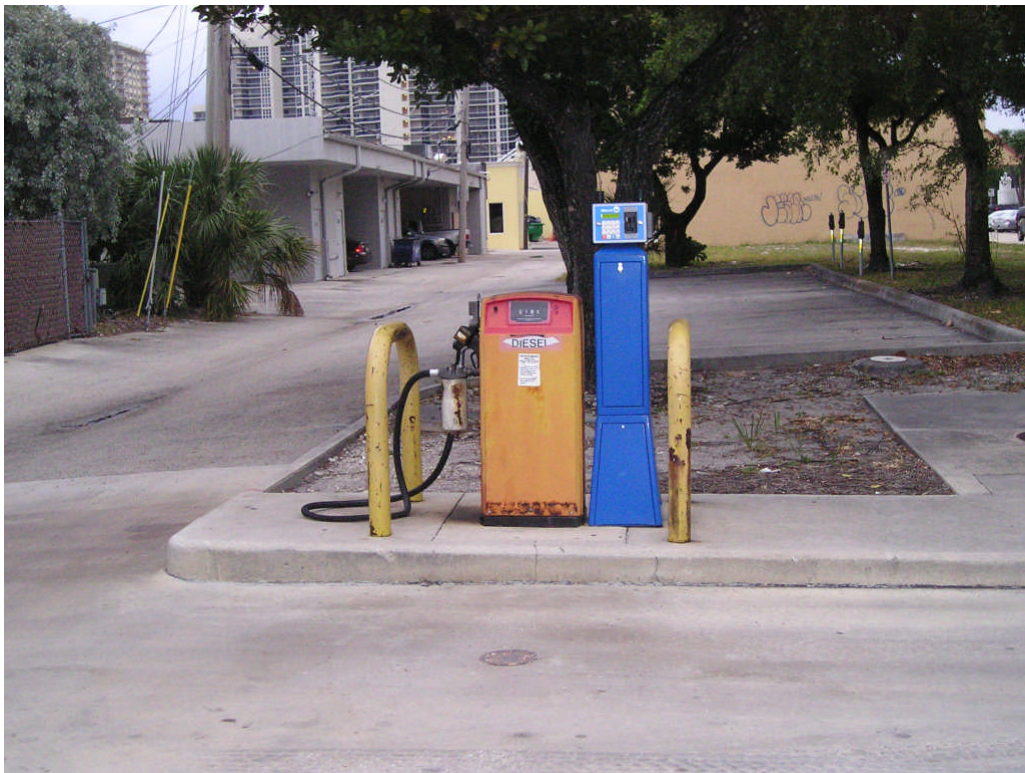
VIEW EASTERLY OF FUEL PUMP AND EXCESS LAND FROM SOUTH SIDE DRIVEWAY
