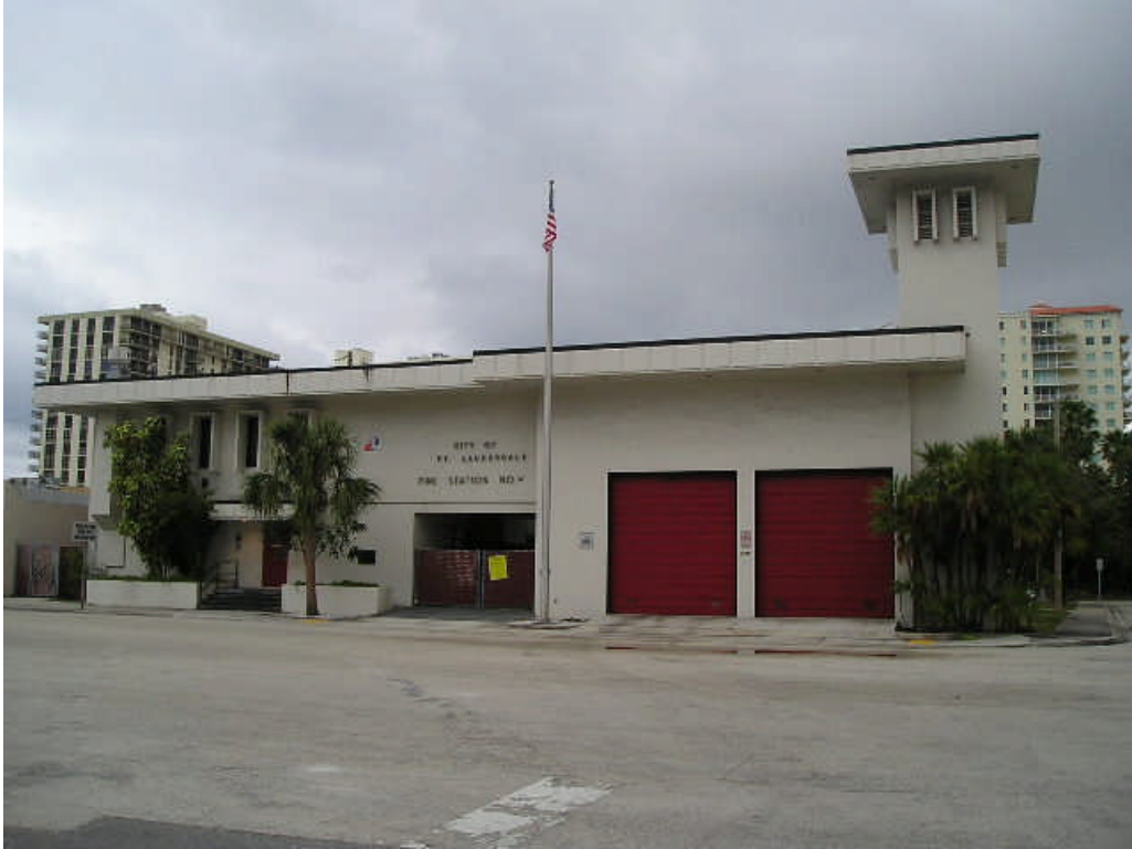
VIEW SOUTHERLY FROM ACROSS NE 32 ST.
