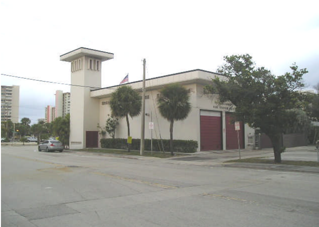
VIEW NORTHEASTERLY OF SUBJECT PROPERTY
