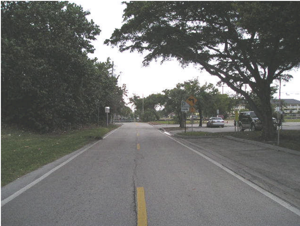
VIEW WESTERLY ALONG ACCESS ROAD
