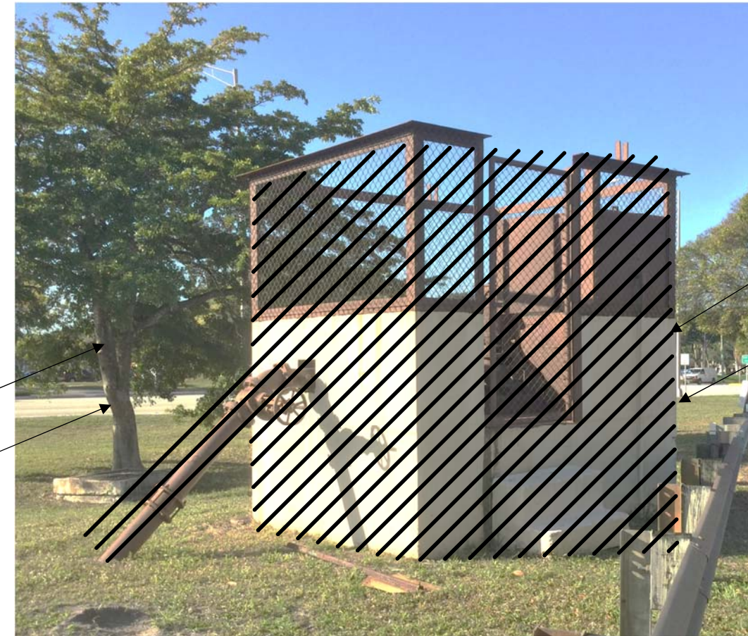
DEMOLITION PHOTO – PW-3 NTS
