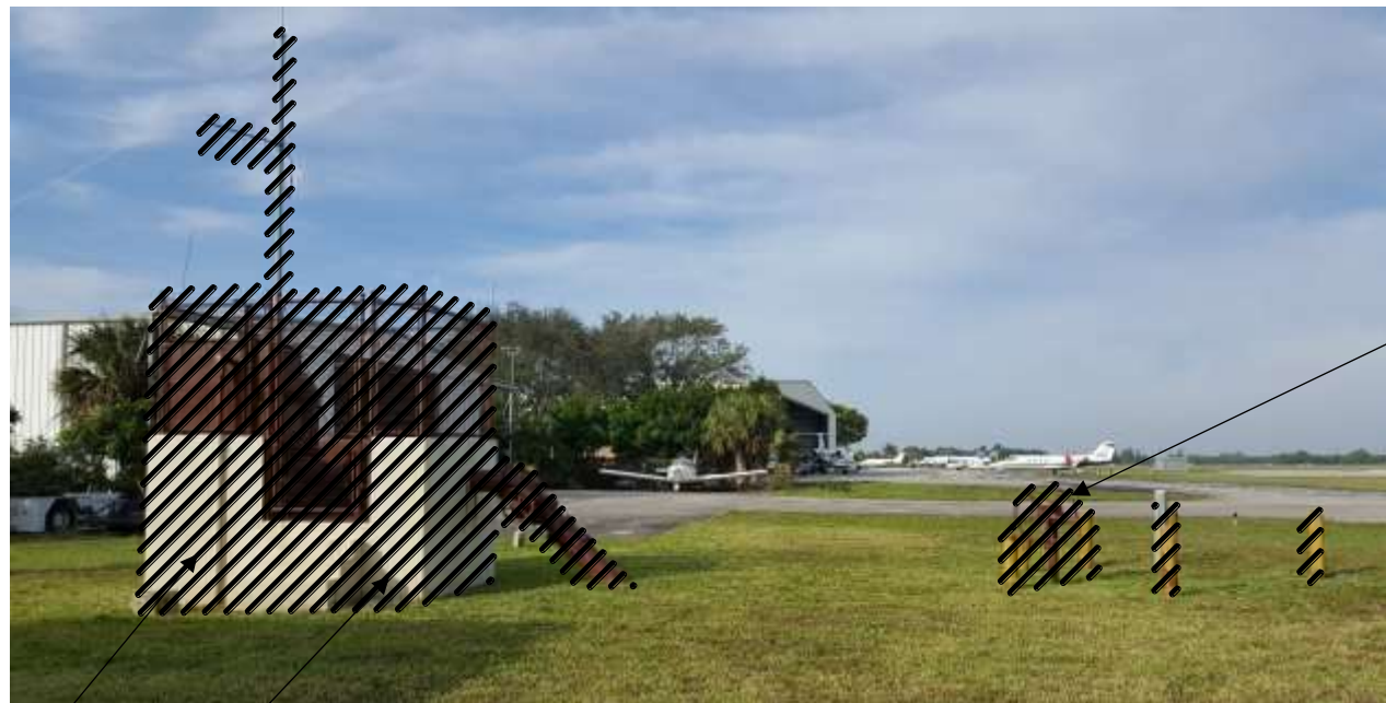
DEMOLITION PHOTO – PW-21 NTS
