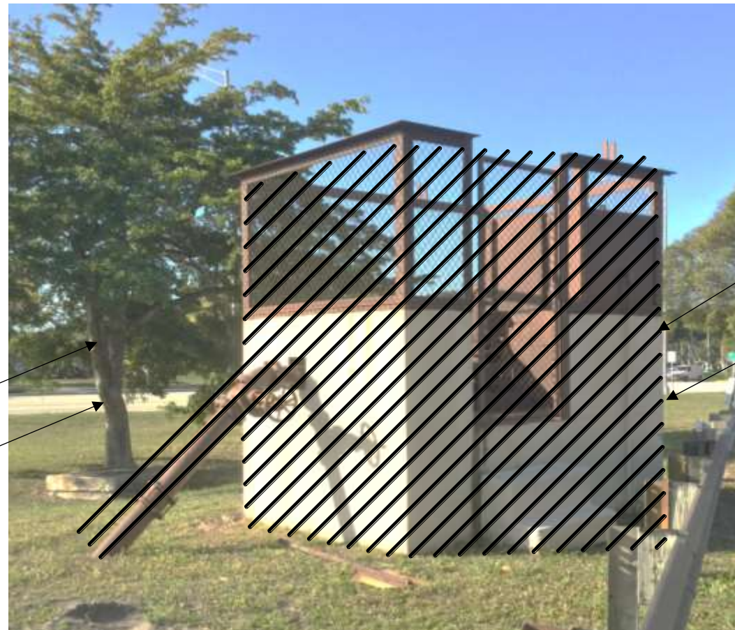
DEMOLITION PHOTO – PW-3 NTS
