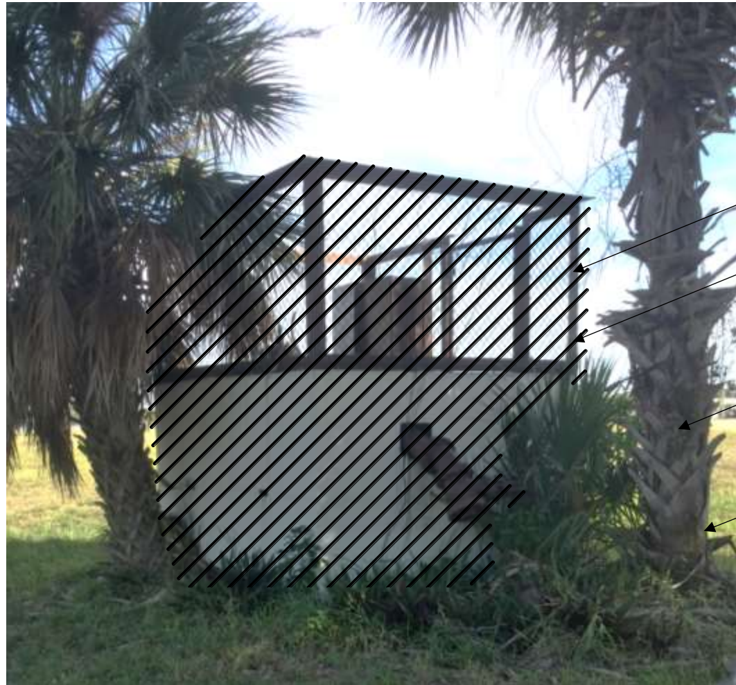
DEMOLITION PHOTO – PW-7 NTS
