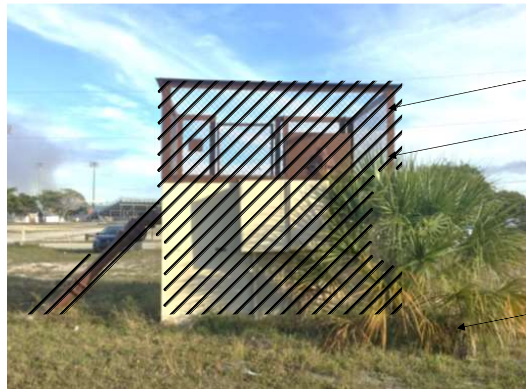
DEMOLITION PHOTO – PW-8 NTS
