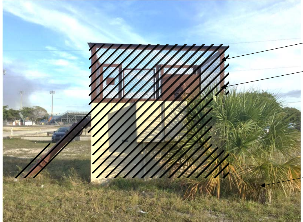
DEMOLITION PHOTO – PW-8 NTS
