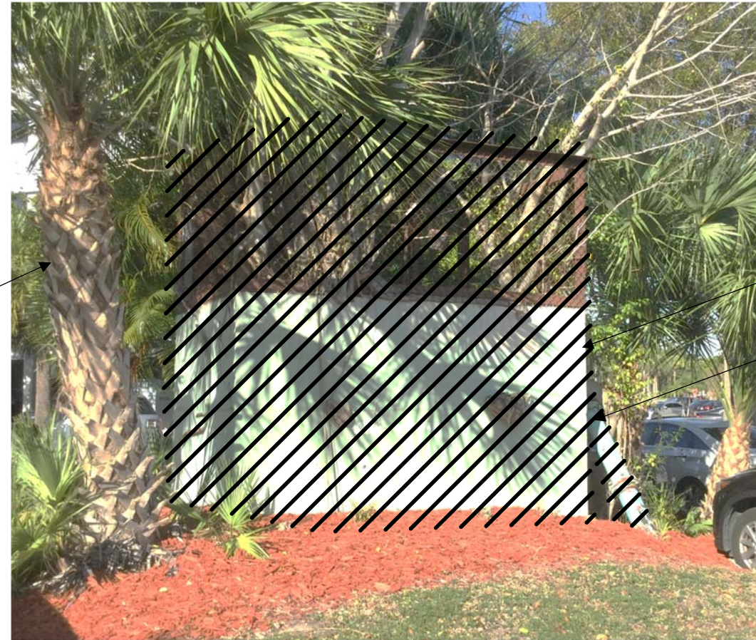
DEMOLITION PHOTO – PW-2 NTS
