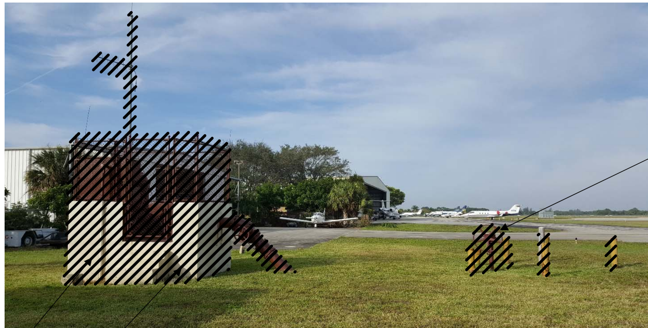
DEMOLITION PHOTO – PW-21 NTS
