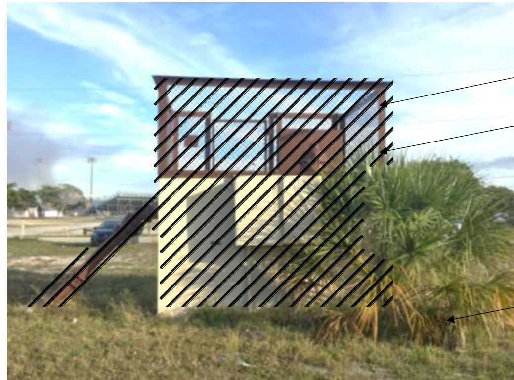
DEMOLITION PHOTO – PW-8 NTS
