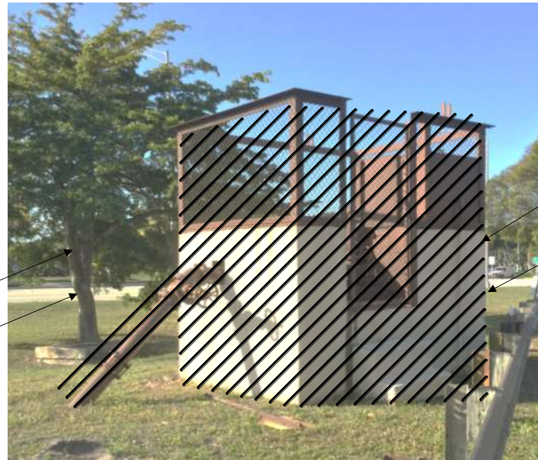
DEMOLITION PHOTO – PW-3 NTS
