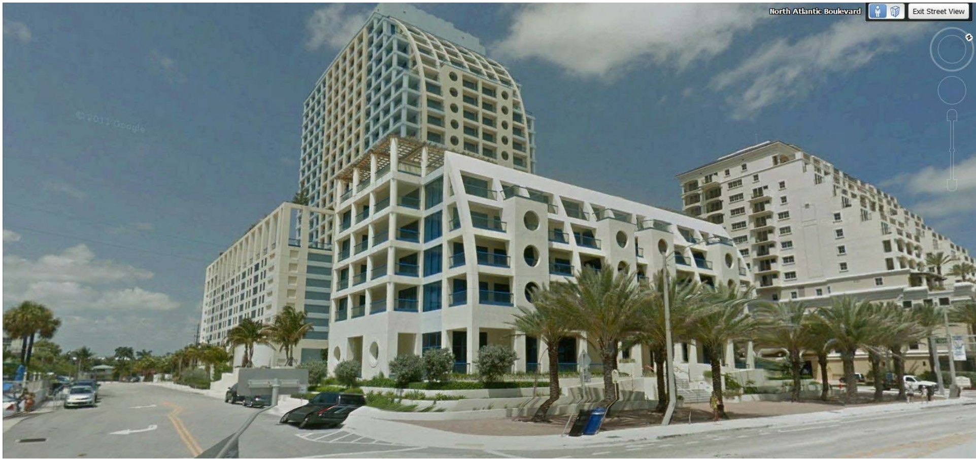
EXISTING VIEW CONNER OF WINDAMAR AND N ATLANTINC BOULEVARD 2 A-45
