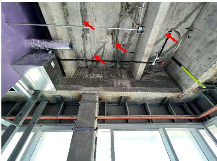
Figure 33. Example of cracks (see red arrows) in the reinforced concrete slab (at the roof) which have been repaired
