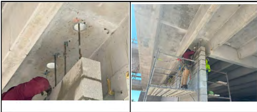
Figure 20. Photographs from Threshold Inspection Report No. 099 showing issue noted by inspector at top of "HQ Level 3 South CMU wall". Note PTA anchors and connection of vertical masonry bars to above slab in left image. Note that the bars are generally spliced to anchors attached to the slab with screws
