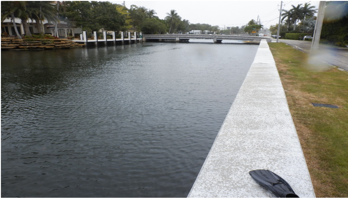
1. Northern portion of the subject site, facing south along the canal.
