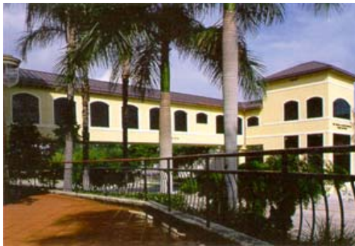
Elevated Skywalk Broward Center for the Performing Arts
