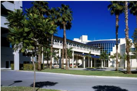
Memorial Hospital West MOB & Parking Garage Pembroke Pines, FL
