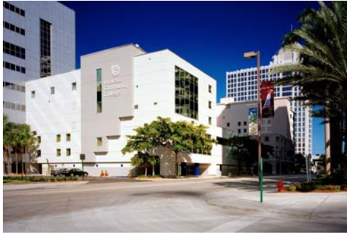
Façade Renovation of Broward College Phase III Downtown Campus
