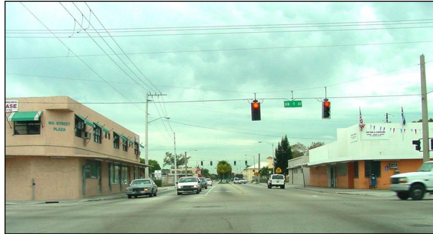
Figure 3.4, Sistrunk/NW 6 th Street Prior to Corridor Improvements
