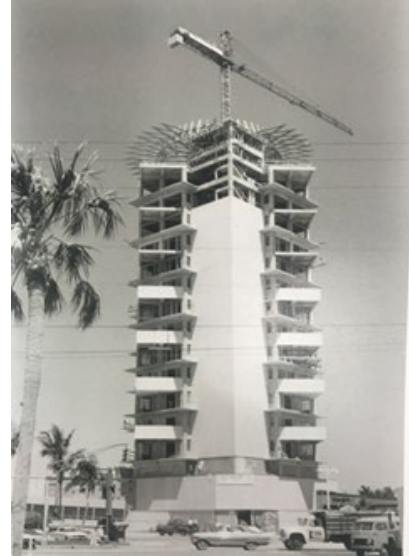
Pier 66 Hotel Tower during Construction, Source: Fort Lauderdale Historical Society.
