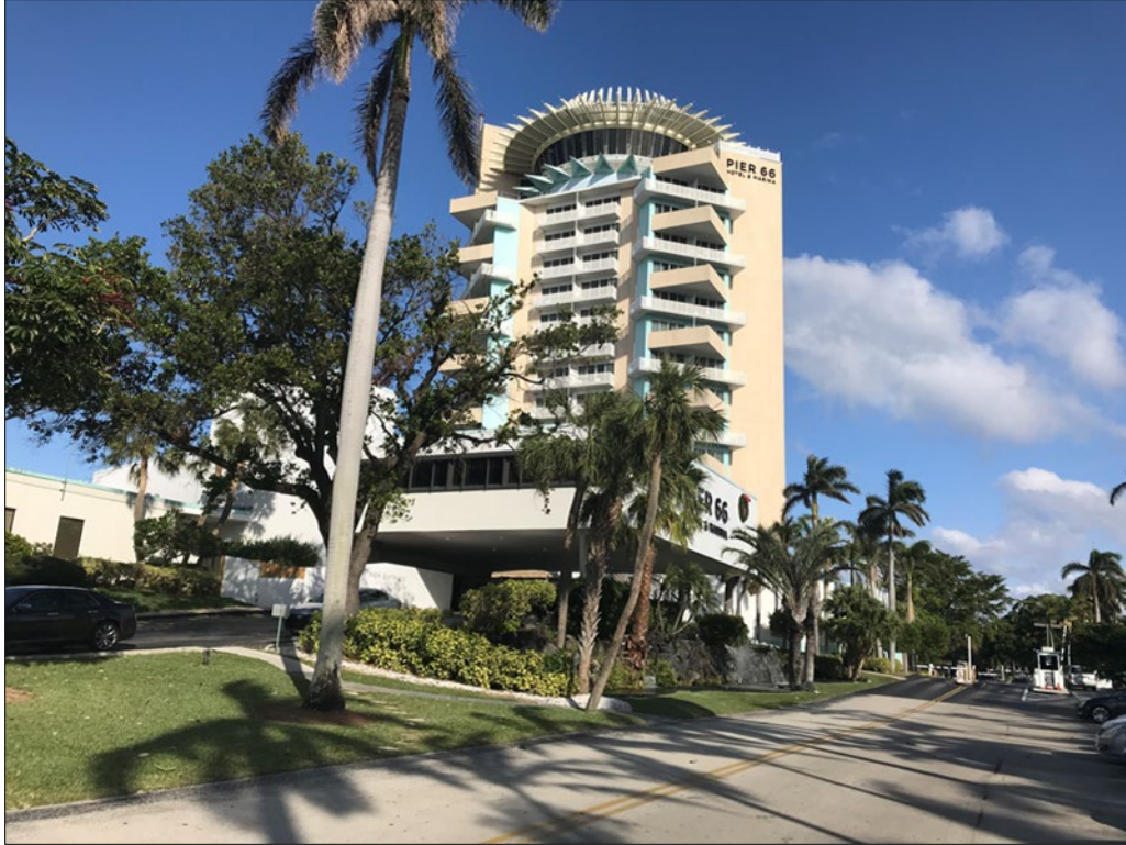
Figure 3. Pier 66 Hotel Tower. Southwest building perspective and site, camera facing northeast. Photograph taken January, 2018.
