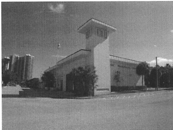
North and West Elevations
