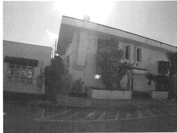
Looking Southwest at East Elevation
