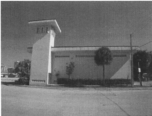
Looking East at West Elevation
