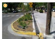
17 Curb Extension with Chase Cover. Source: NACTO
