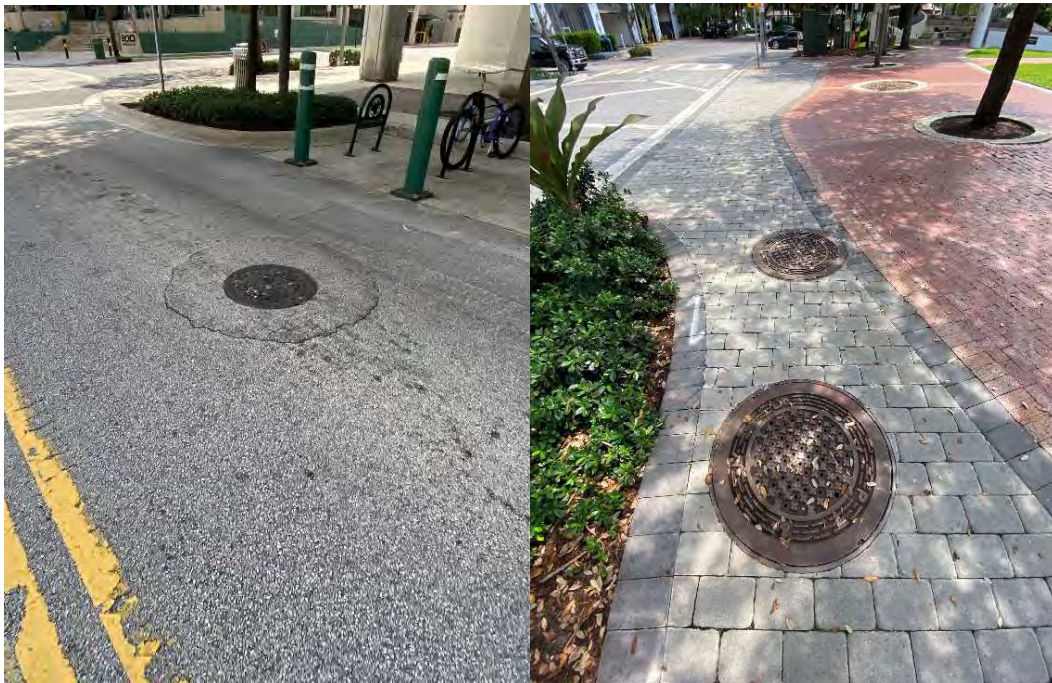
Existing utilities in center of travel lane and sidewalk area
