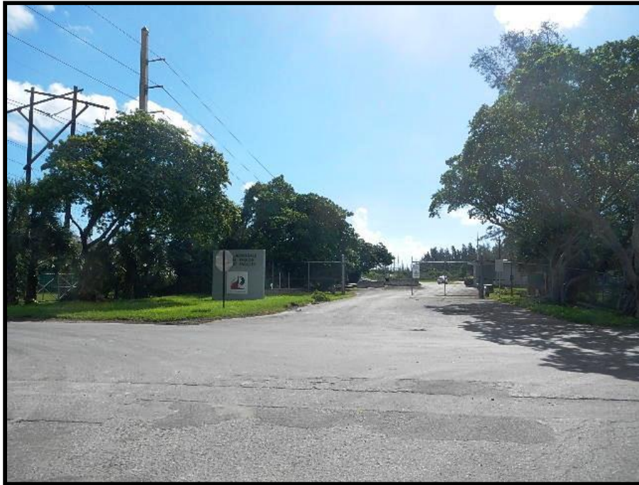
Above: 1. View looking east into site along entrance drive.
