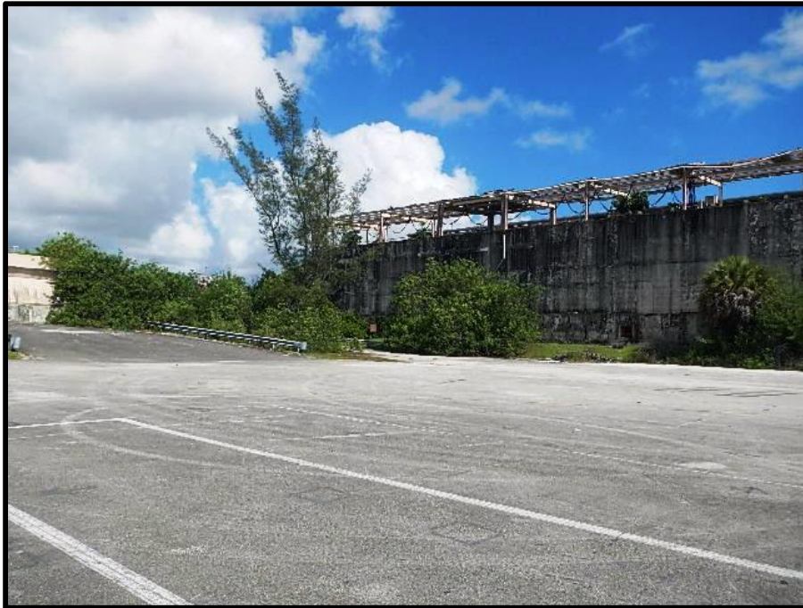
Above: 7. View obsolete equipment on the site.
