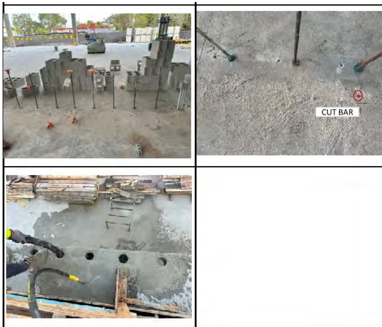
Figure 16. Photographs from Threshold Inspection Report No. 073 showing bars doweled 3 inches into slab-on-ground after original bars were mislocated (top photographs), and filling of grouted cells (bottom photograph)
