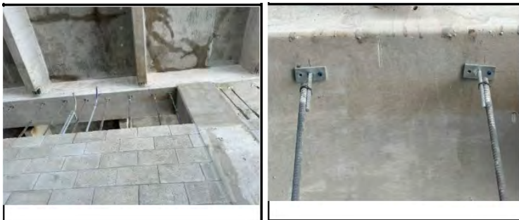
Figure 26. Photographs from Threshold Inspection Report No. 123 showing PTA connectors at bottom of soffit beam with only one screw attaching the plate of the anchor to the soffit beam
