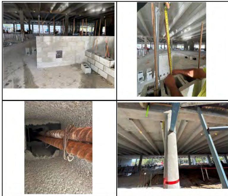
Figure 18. Photographs from Threshold Inspection Report No. 084. Upper photographs and lower right photograph appear to be of the first story prior to full installation of CMU walls. Note the lack of shoring indicating that the CMU walls were not constructed as bearing walls
