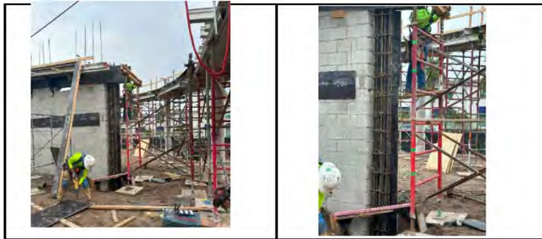
Figure 23. Photographs from Threshold Inspection Report No. 105 showing CMU wall in Area E under construction. Since the wall is being constructed prior to the roof structure, this CMU wall will take load from the roof structure as a bearing wall
