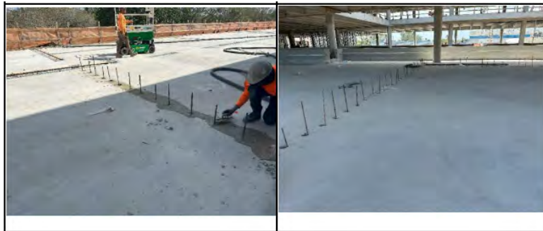
Figure 25. Photographs from Threshold Inspection Report No. 109 showing dowels extending through cored holes in slab. These dowels appear to be from the CMU wall below
