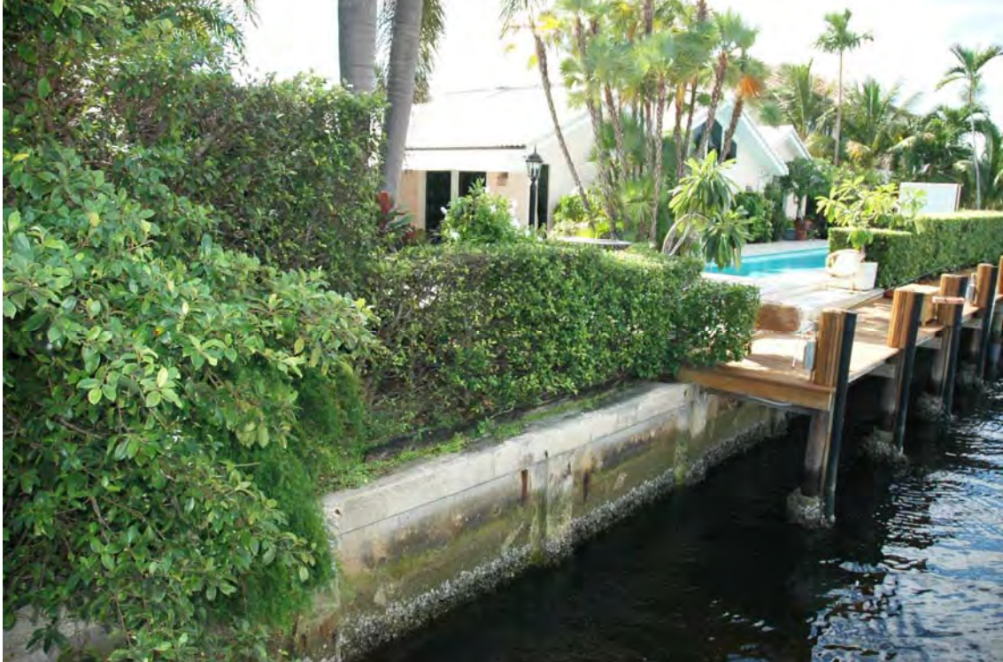
1. Western property boundary, facing southwest along the canal.
