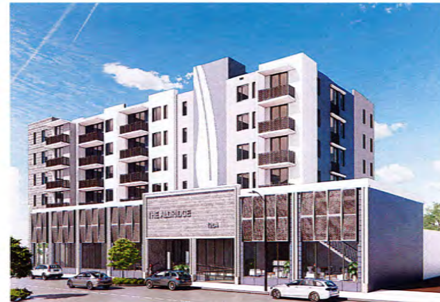
NORTH WEST VIEW
