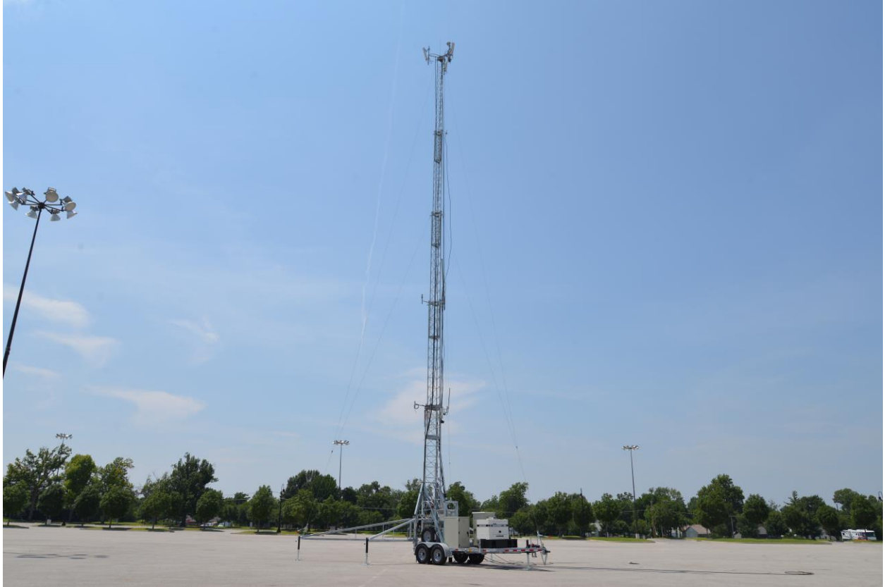
Alltech Tower Deployed In Parking Lot
