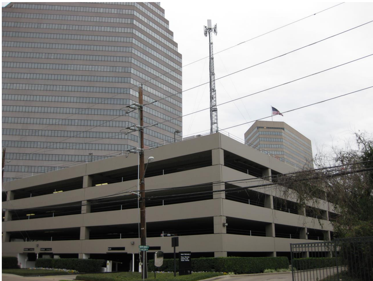
ATC-106 Tower Trailer On Top of Parking Garage
