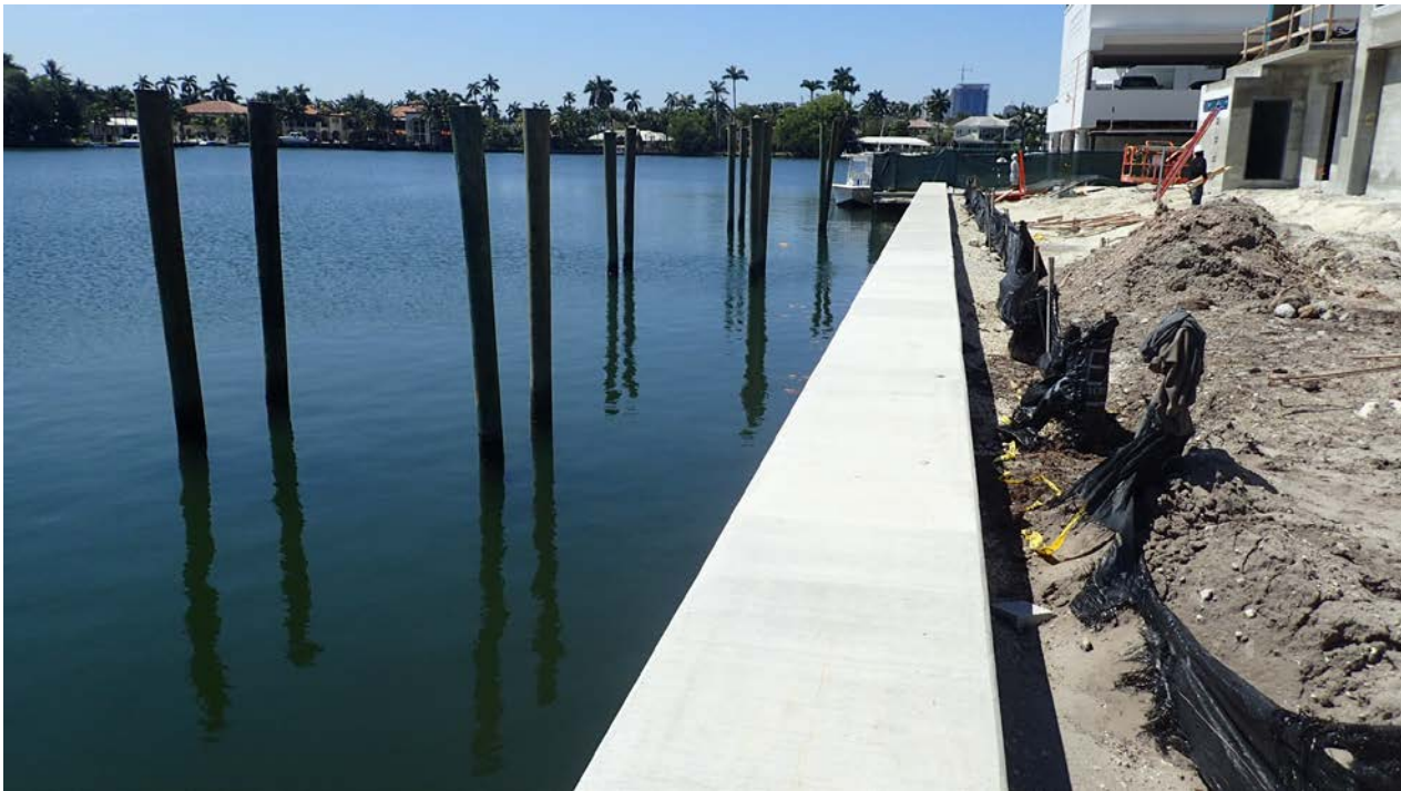
2. East corner of the subject site, facing west.
