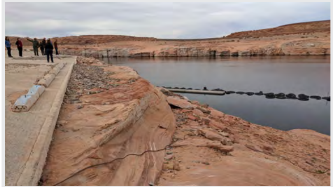
End of Antelope Point Launch Ramp several feet above lake level
