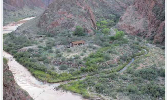
View of the wastewater reclamation facility from Trail 3 at Grand Canyon National Park, Arizona
