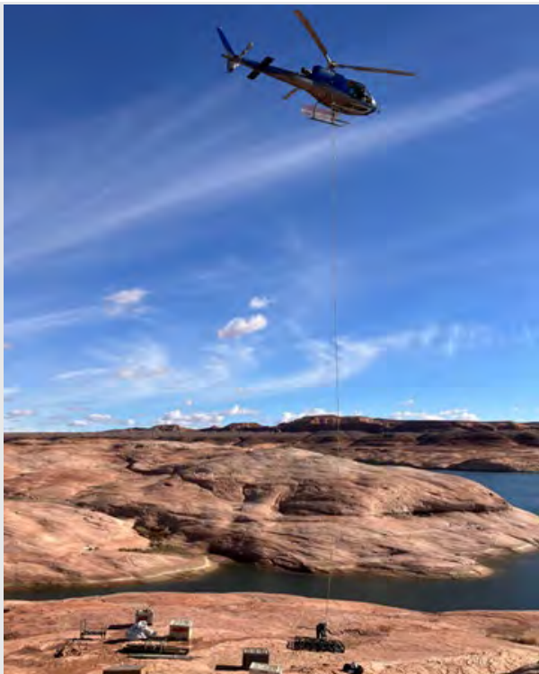
Helicopter delivering equipment to site for geotechnical investigation at proposed launch ramp location for Bullfrog
