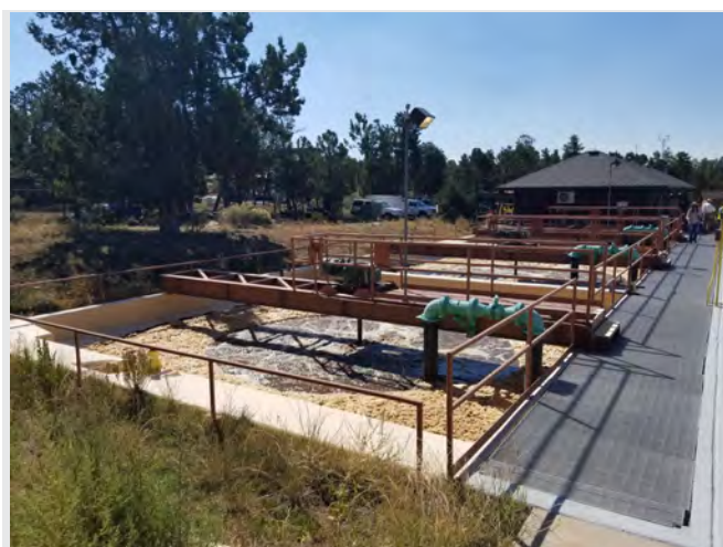
Existing Aeration Basins at South Rim WWTP
