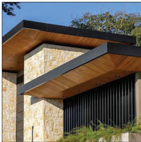
06 - WOODEN ROOF SOFFIT
