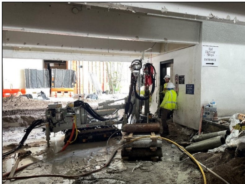
Photo : Low headroom Micropile drill rig
