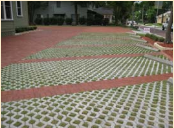
[Figure 4.265] A Porous or permeable pavement is highly effective when applied to parking spaces.
