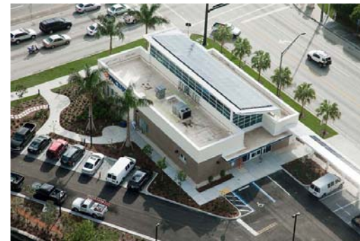
[Figure 4.267] This bank in Fort Lauderdale is one of several LEED Certified buildings in the City.
