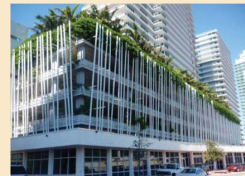
[Figure 4.254] A parking garage with sophisticated styling, screening, windows and green roof elements integrated into the design.
