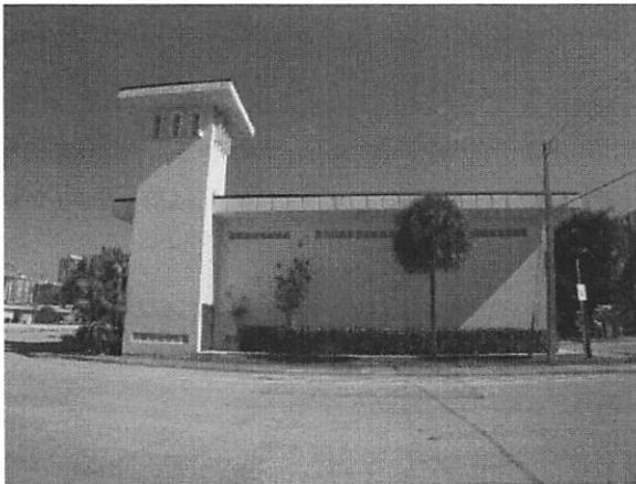
Looking East at West Elevation
