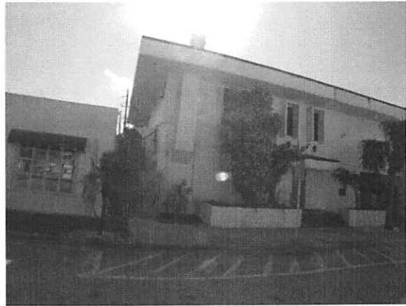
Looking Southwest at East Elevation
