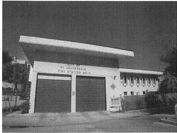
Looking Northeast at Building Rear
