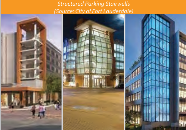
Figure 5.16: Structured Parking Stairwells
