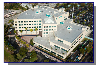
Broward Sheriff’s Office Public Safety Building Renovation/Hardening
