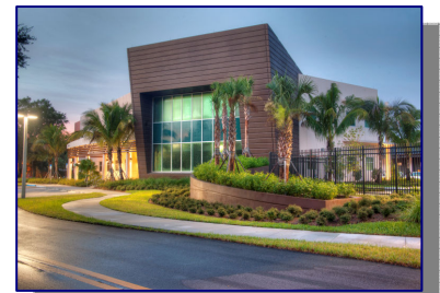
Coconut Creek New Public Works Building
