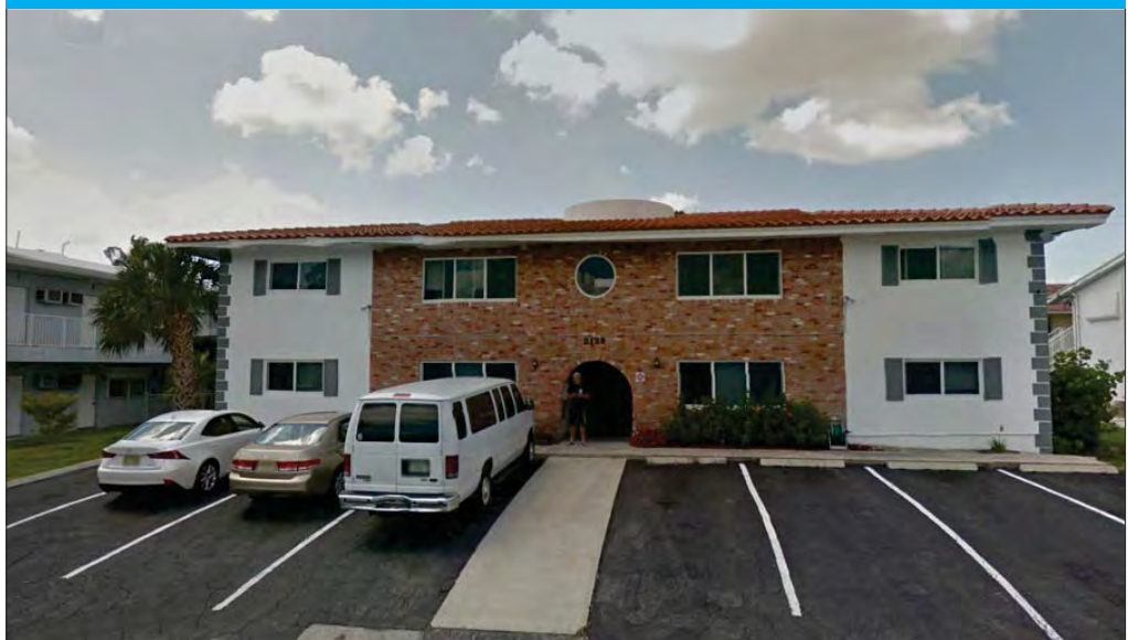
Figure 14: Fort Lauderdale Apartment Building Turned Into a Recovery Mini-Institution
