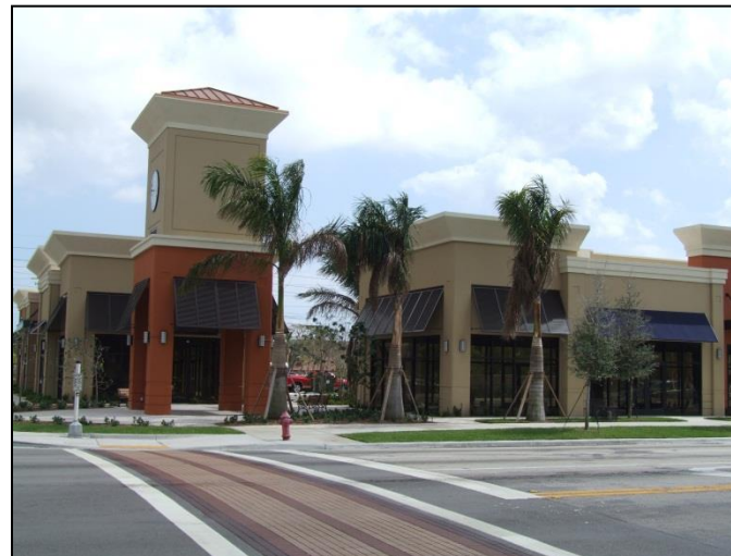
Figure 3.6, Sistrunk Boulevard/NW 6 th Street after Corridor Improvements
