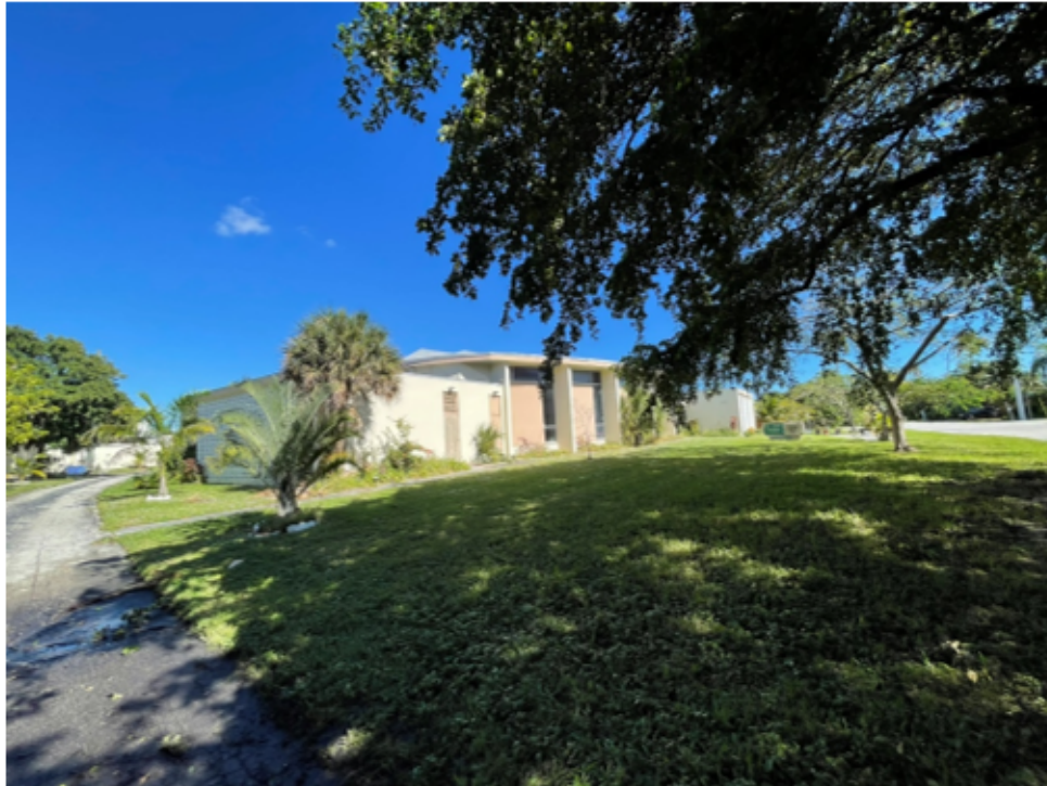
FRONT VIEW OF SUBJECT FROM 19 TH STREET
