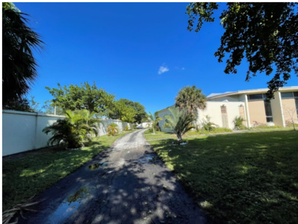
FRONT VIEW OF SUBJECT FROM 19 TH STREET
