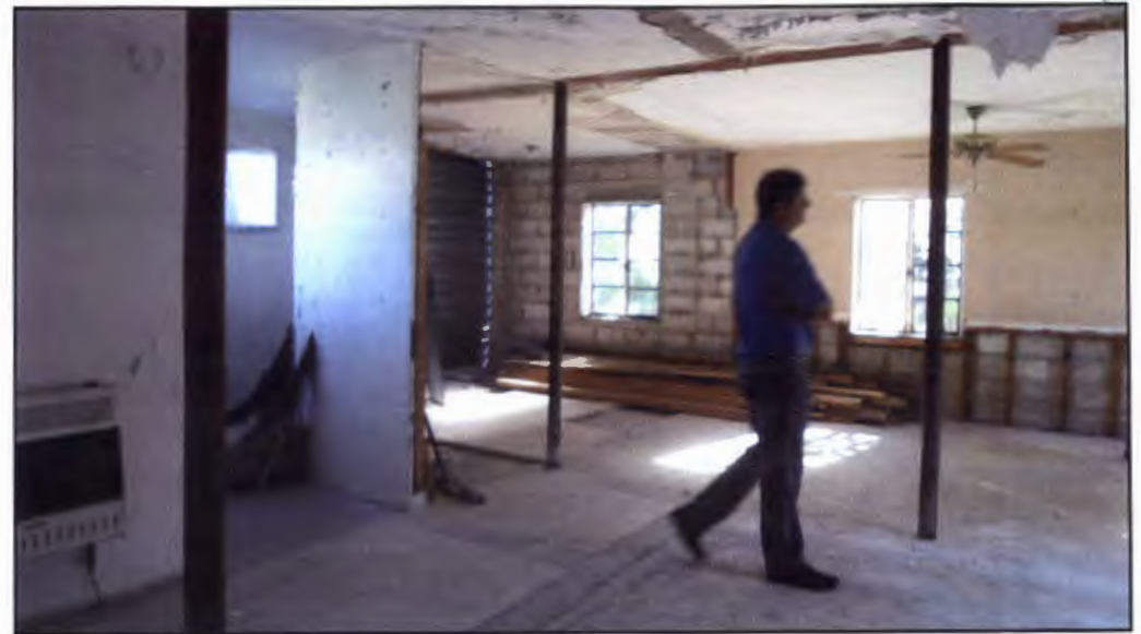
Interior with required supports to hold up roof
