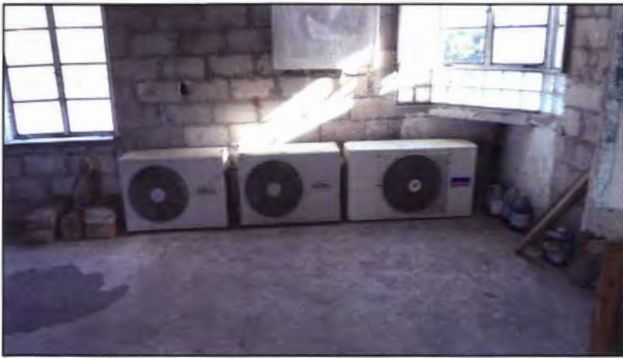
Block construction- not poured as previously stated
