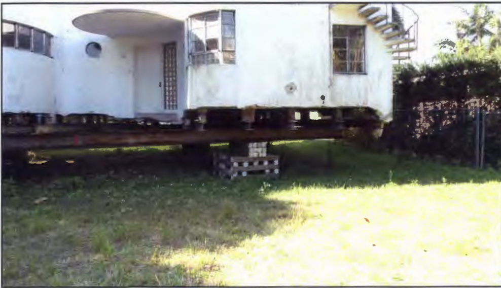
Unsafe stairs and all around wall cracking and rusting
