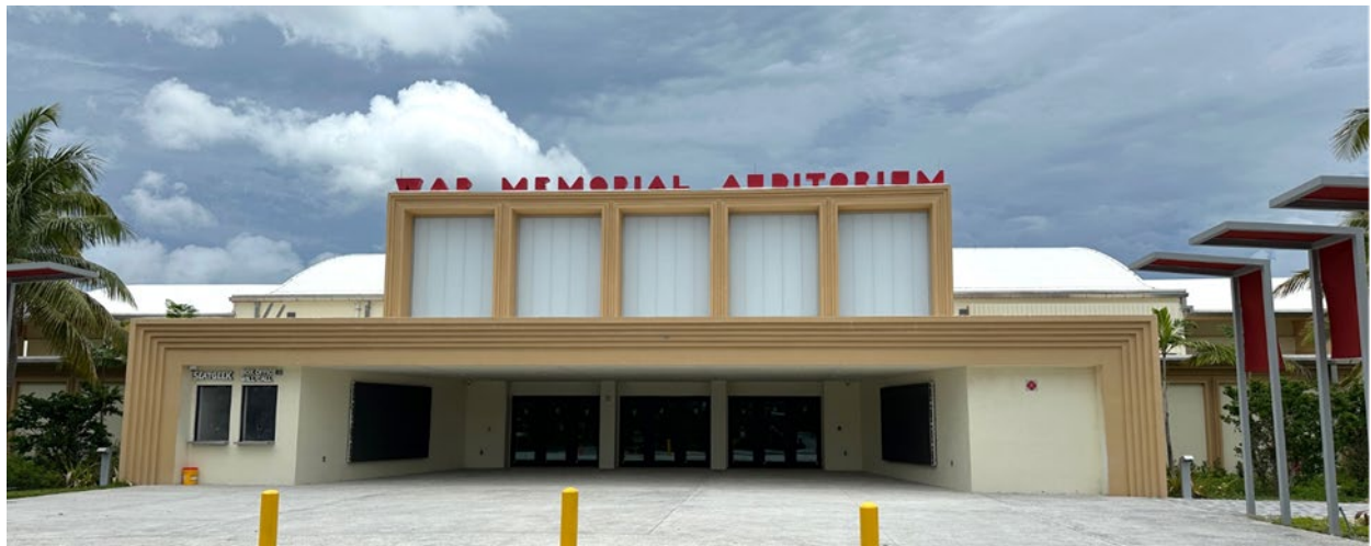
Photo of Existing War Memorial Auditorium
