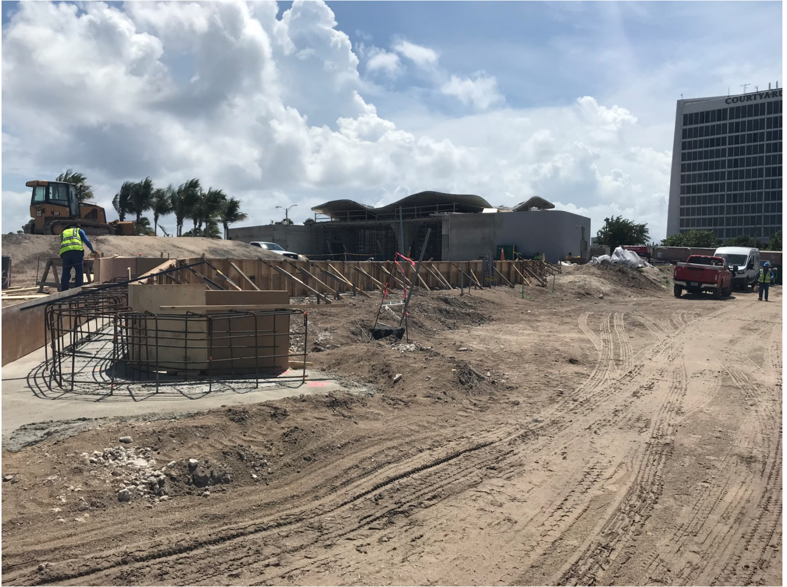
OCEANSIDE PARK PROGRESS PHOTO TAKEN ON 9-12-2019 (CAST-IN-PLACE SITE WALL FORMWORK AND FOUNDATION)
