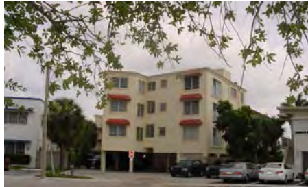
(East of 425 Bayshore Drive) 3-story residential over parking
